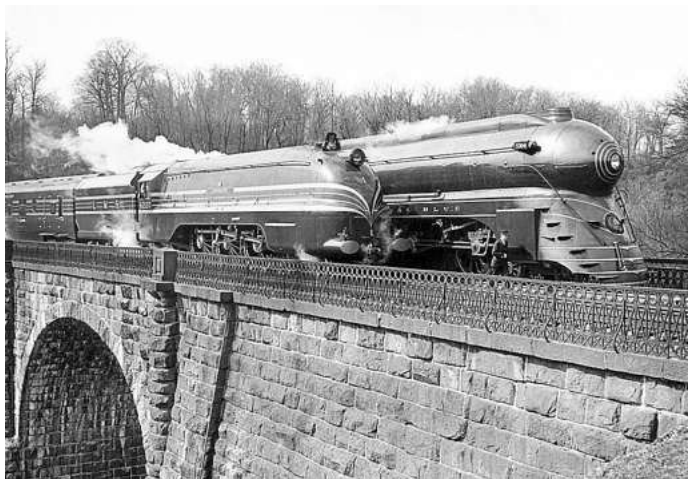
Returning from Washington DC to Baltimore on its March 18, 1939, press trip, the 'Coronation Scot' was stopped on the Thomas Viaduct over the Patuxent River near Relay, Maryland. Built in 1835, it is said to be the world's oldest stone railway viaduct. 'Coronation' was posed for press pictures alongside the Baltimore & Ohio Railroad's 'Capitol Limited' headed by streamlined P7 Pacific No. 5304.
