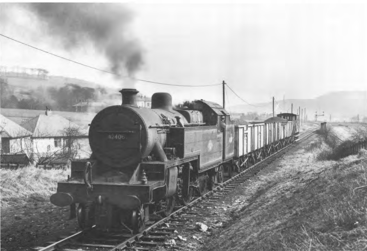
Below: Mirfield's Fowler 2-6-4T No. 42406 propels the 10.10am Newtown - Hillhouse P96 trip towards Red Doles Junction at 10.16 on 23rd March, 1963. Propelling was the normal practice in order to negotiate Red Doles junction without running round.
