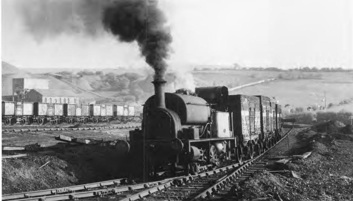
Above: A much older Hudswell Clarke 0-4-0ST, works no. 614 of 1902 shunts a rake of internal wagons in the yard at Emley Moor Colliery at 07.49 on 12th May, 1965. Internal rail traffic continued for a few months in 1983 after the Clayton West branch closed.
