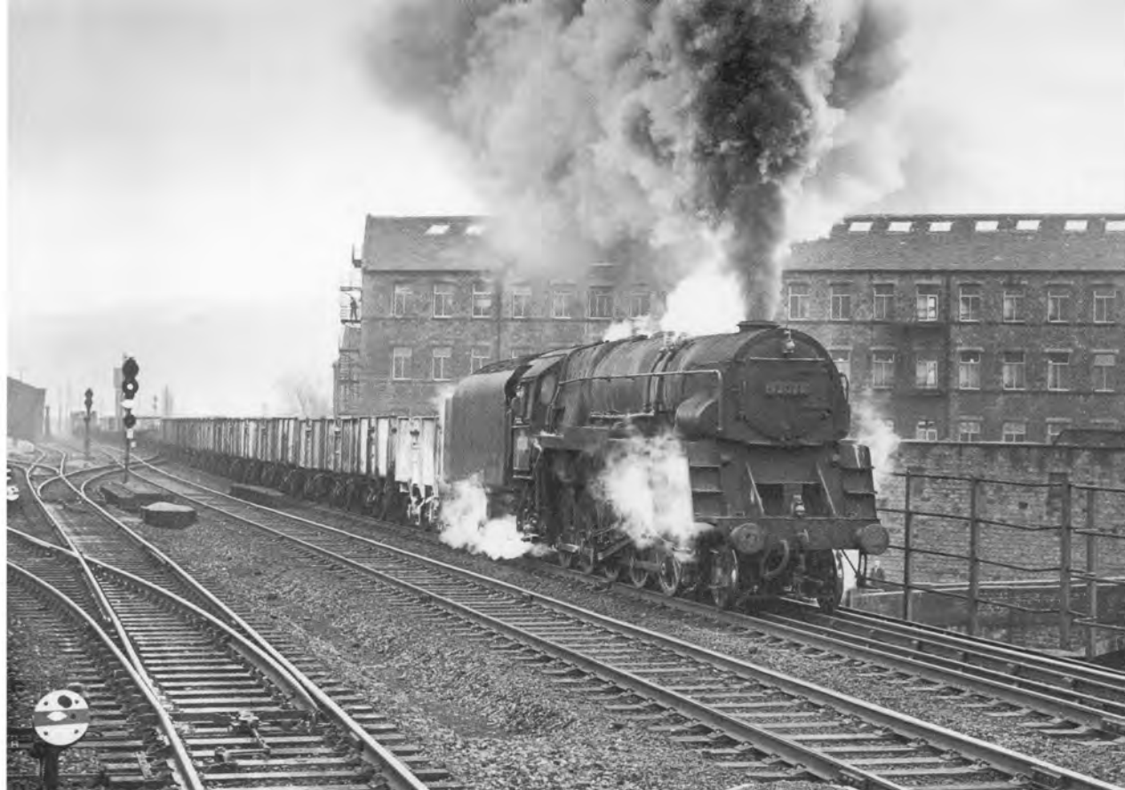
Above: How we miss sights like this! Former Crosti boilered 9F 2-10-0 No. 92026 makes a volcanic recovery from a signal check alongside Mirfield station while working a long drag of westbound empties at 12.45 on 2nd February, 1965. Alongside the train is a searchlight signal connected with the speed signalling system, of which more detail is given in Railway Memories No.11 .
