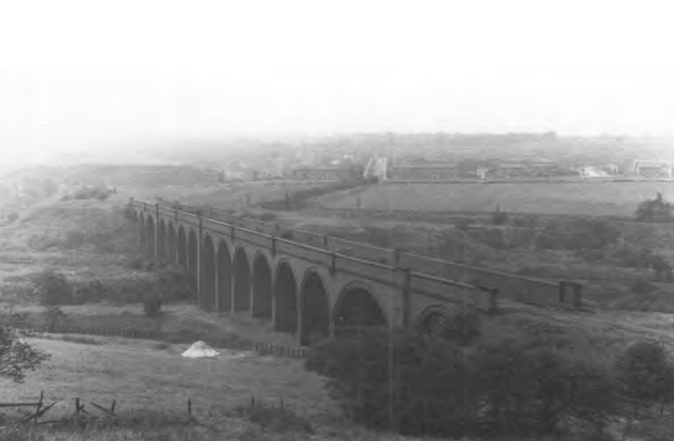
Above: The 15-arch brick viaduct carrying the Mirfield-Red Doles section of the Newtown branch over the Colne Valley at Bradley. This view, looking towards Huddersfield, was taken in July, 1961, 24 years after the line had been abandoned.
