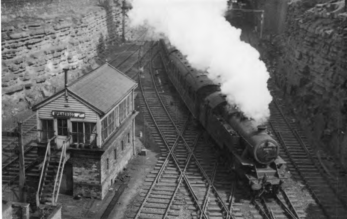
Above: Sandwiched in the rock cutting between Springwood and Gledholt tunnels is Springwood Junction where the Penistone line parts company from the Standedge route and thrusts out through the cutting side onto the lofty heights of Paddock Viaduct. Here, Fairburn 2-6-4T No. 42072 heads a Penistone-bound train, probably from Bradford, past Springwood Jn. signal box which was abolished in 1961 when Huddersfield power box control area was extended.
