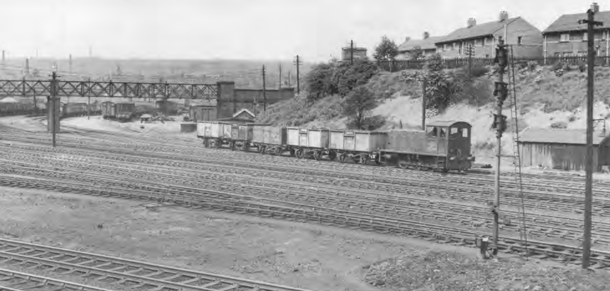
Above: A view of Hillhouse sidings with Drewry 204hp 0-6-0 diesel shunter No. D2266 at work in May, 1960. Crossing the scene is the footbridge leading to the engine shed while the freight terminal is through the right hand span of the bridge. The roads in front of the train lead to the locomotive depot and sorting sidings.
