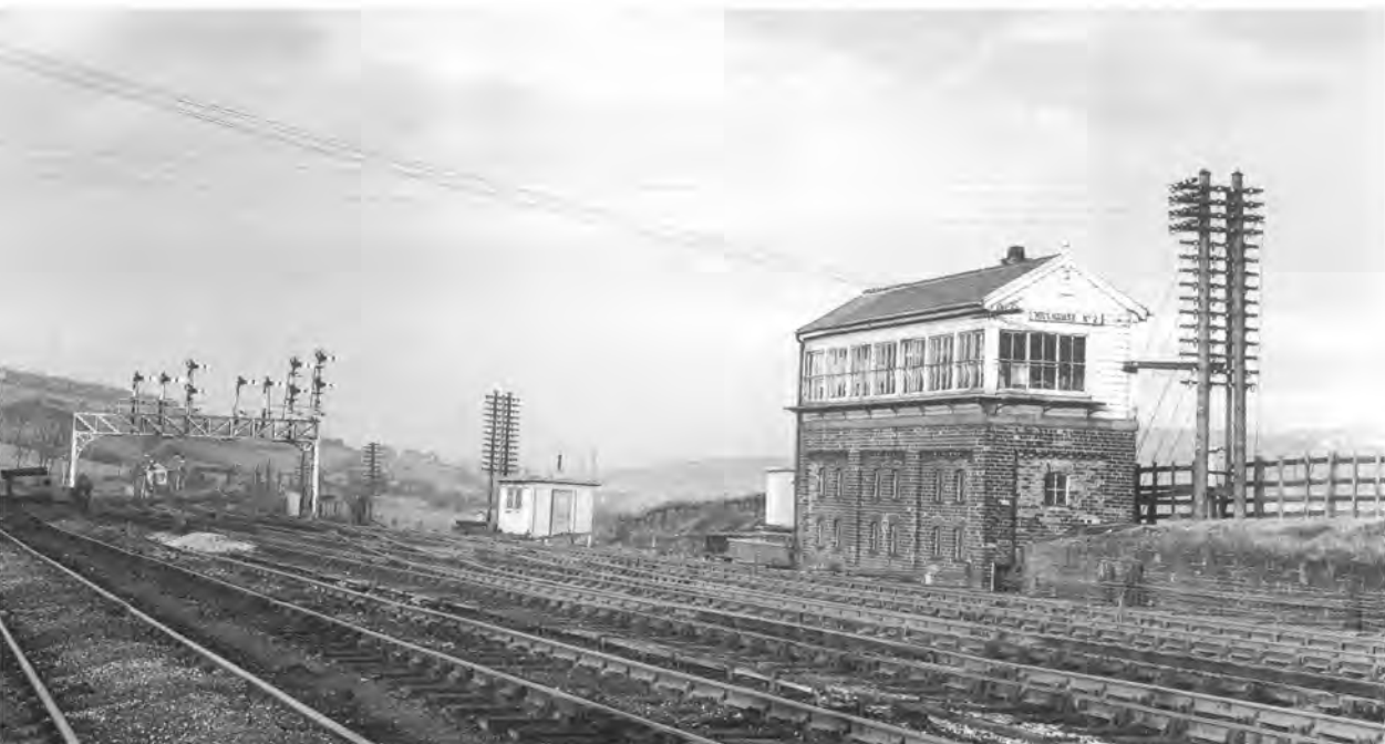
Hillhouse No.2 signal box on 24th April, 1965 looking north towards the fine gantry protecting the approach to Huddersfield. The box in the distance through the gantry is Red Doles, junction with the Newtown branch. Beyond that an overbridge marks the abandoned Midland line from Mirfield. Back in 1957 Hillhouse No.2 box was open continuously whereas Red Doles was open as required.
