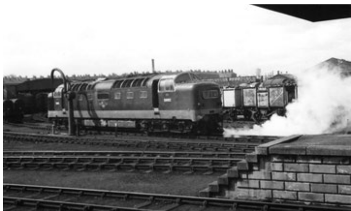
At York, D9002 blows off steam from its train heating boiler. JOHN DYER
